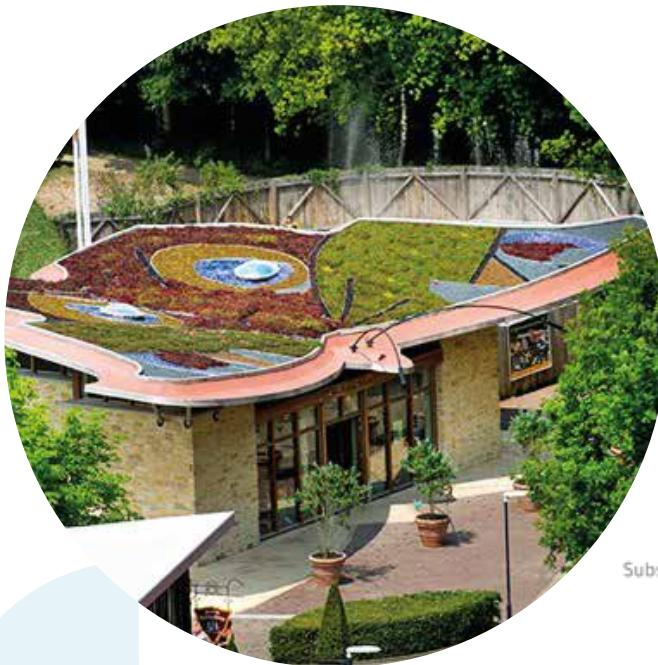
Low-density green roof systems are lightweight roofs consist of a wide range of plants and lawns, which are especially adapted for roofs, even under heavy weather conditions. While increasing the quality of their living spaces, these constructions provide an Environmental friendly, natural look to the roofs.
